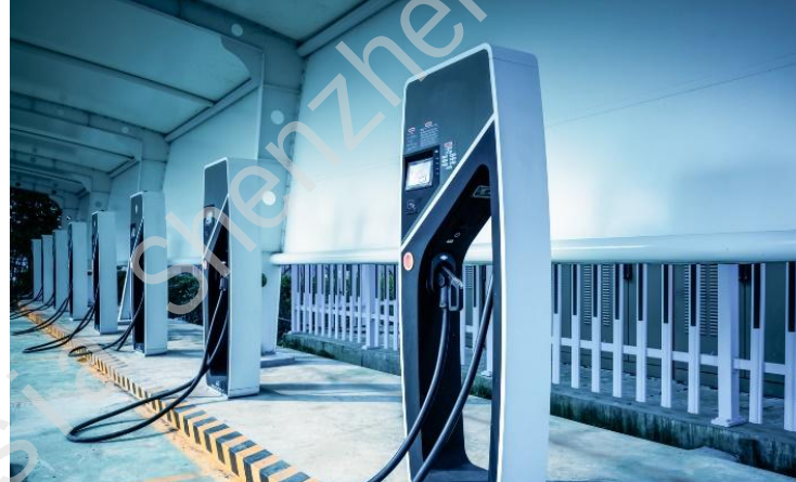
SSCBs, DC Breakers
